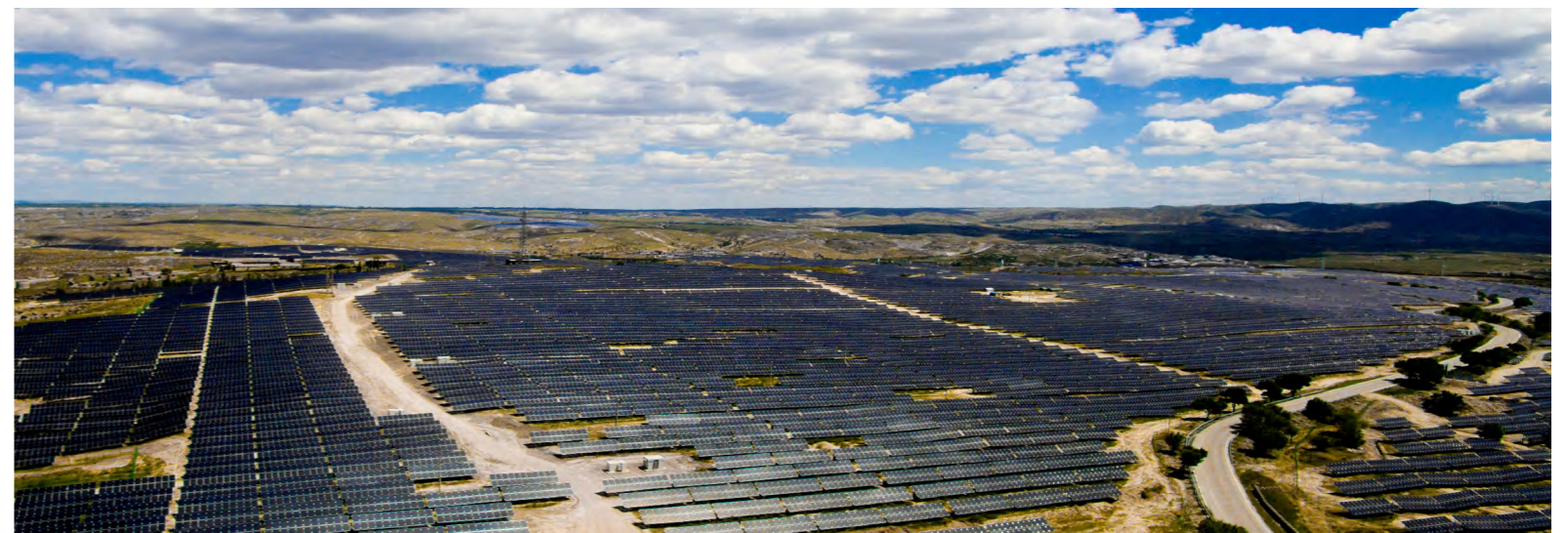
50 MW N-Type bifacial PV plant of national "Top Runner" advanced technology demonstration base in Datong, Shanxi Province, China
